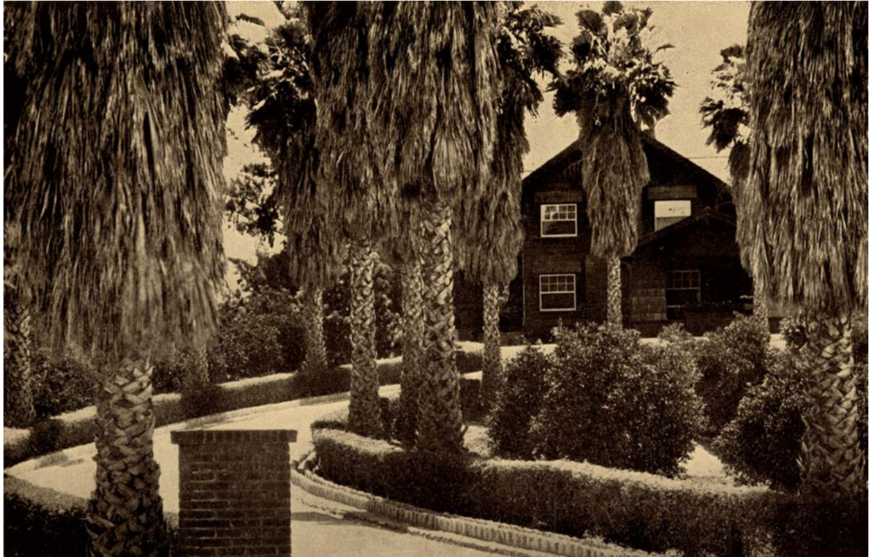
Figure 7. Original driveway and northwest elevation (McDaniel, 1927)
