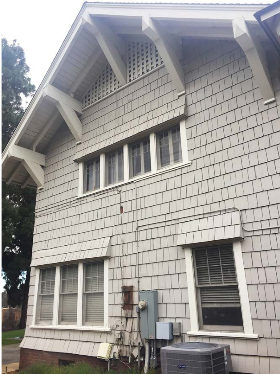
Photo 5. South east elevation. Camera facing west..
